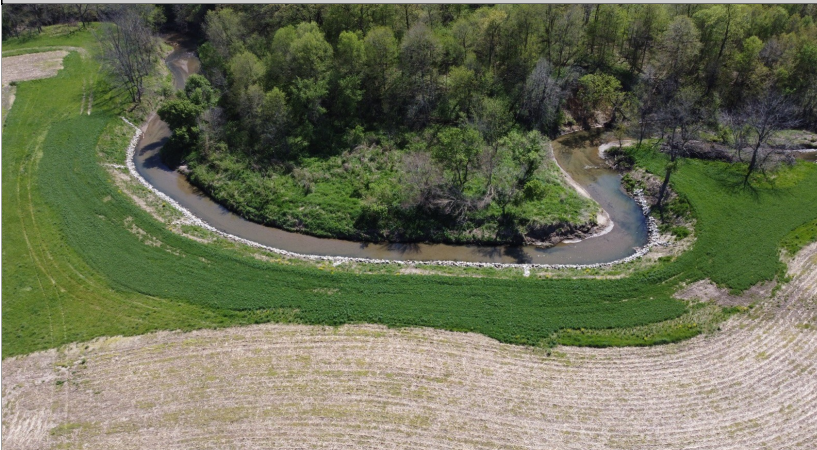
Completed Streambank Stabilization project
