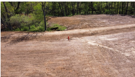
Completed WASCOB project
